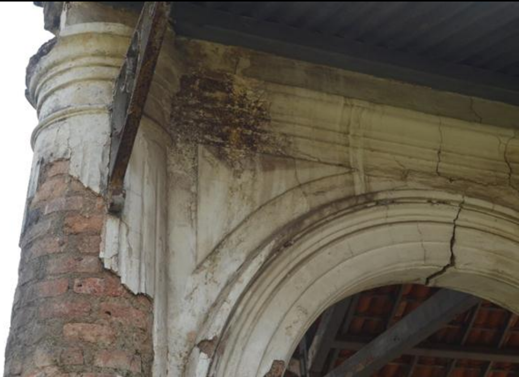
Fig 15. Damaged wall plaster and structural crack due to earthquake and ground shifting
