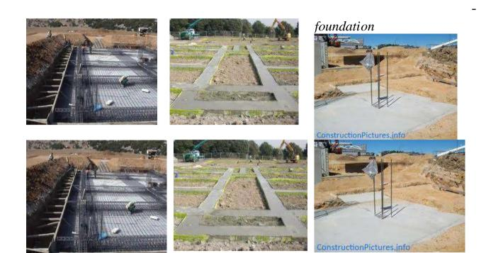
*a)raft foundation b) strip foundation c) pad foundation Figure* 8.1. Types of Foundation
